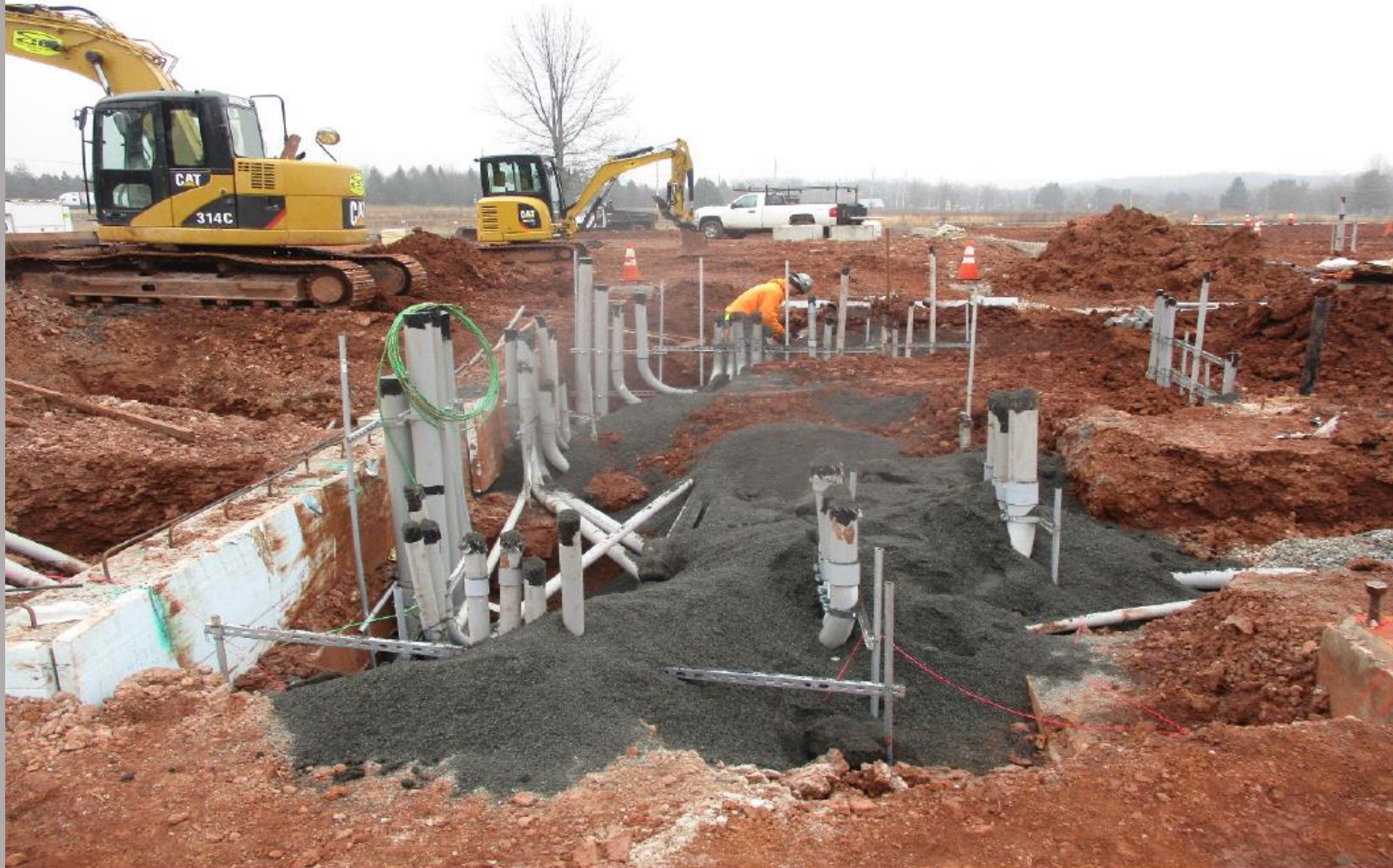
Below Slab Conduit, Electrical Room
