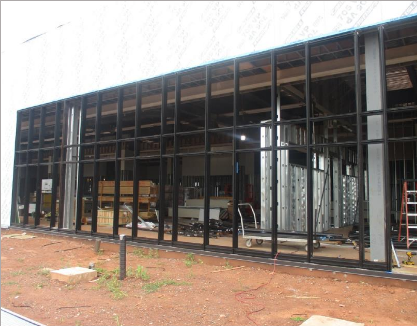
Area B Curtain wall installed
