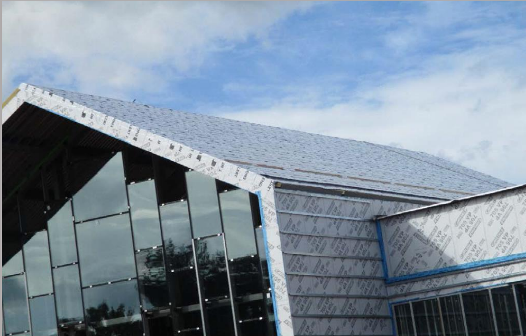
Area "A" Roof to Ice Shield
