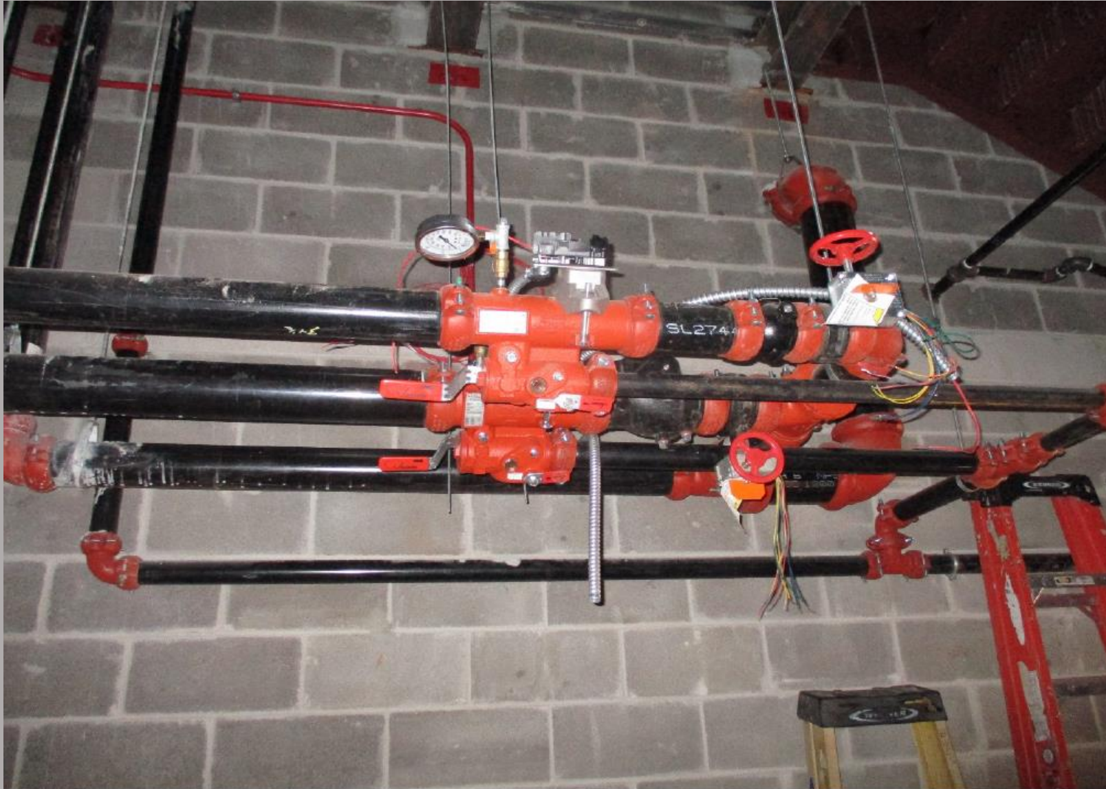
Stairwell C Sprinkler Header
