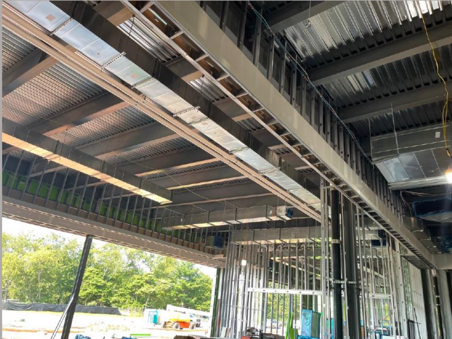
Drywall soffit installation with HVAC installation Area B
