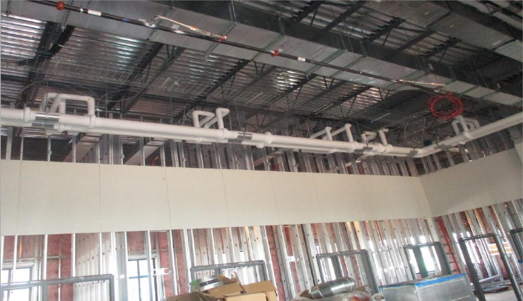
Area "B" Soffit & Pipe Insulation
