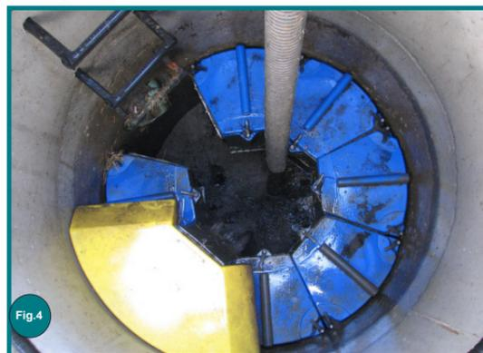
Compliance with your stormwater treatment permit requires using suitable Up-Flo® Filter replacement media bags from Hydro International to ensure the system is functioning as intended (Fig. 2)
