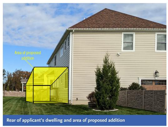
**Description of Addition.** The plans indicate that the addition will extend from the rear of the building, starting 8 inches to the left of the southern facing side wall of the house, extending about 75% of the rear side of the house, and extending back approximately 14 feet. The plan indicates that the area of the addition is 816 sf.
